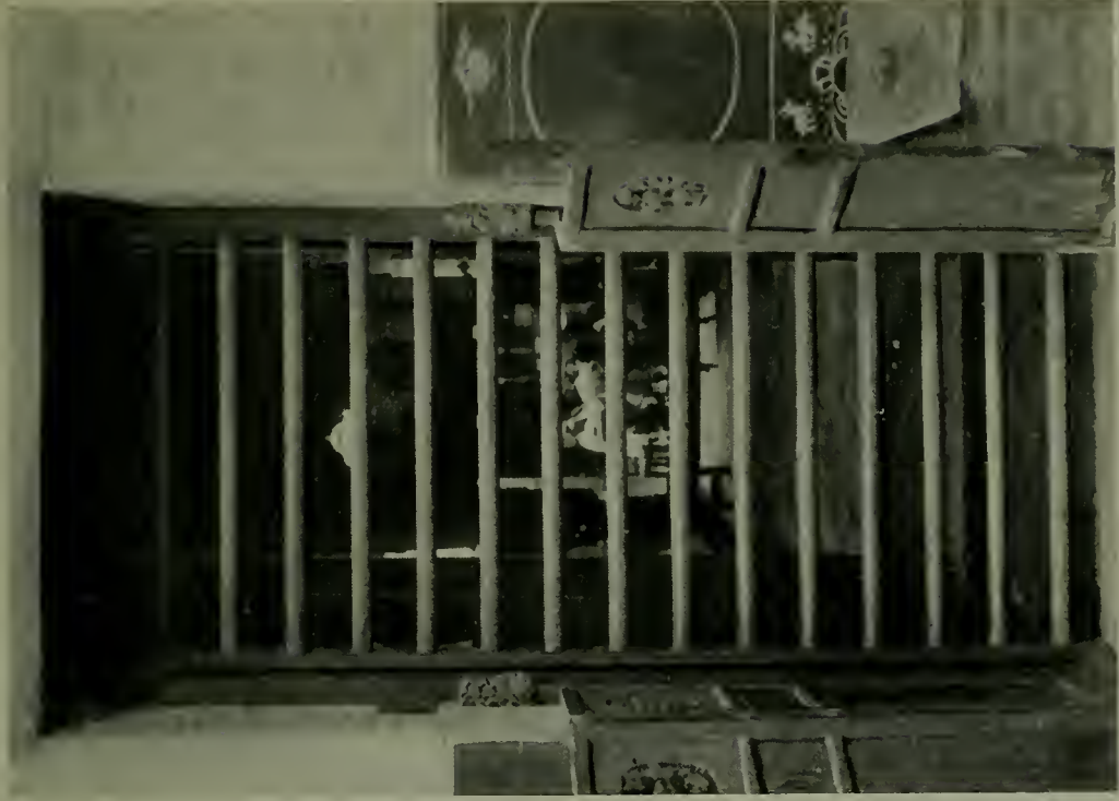
In Canton, where thieves are legion and heat often intense, sliding doors of stout poles protect most well-to-do households and shops
